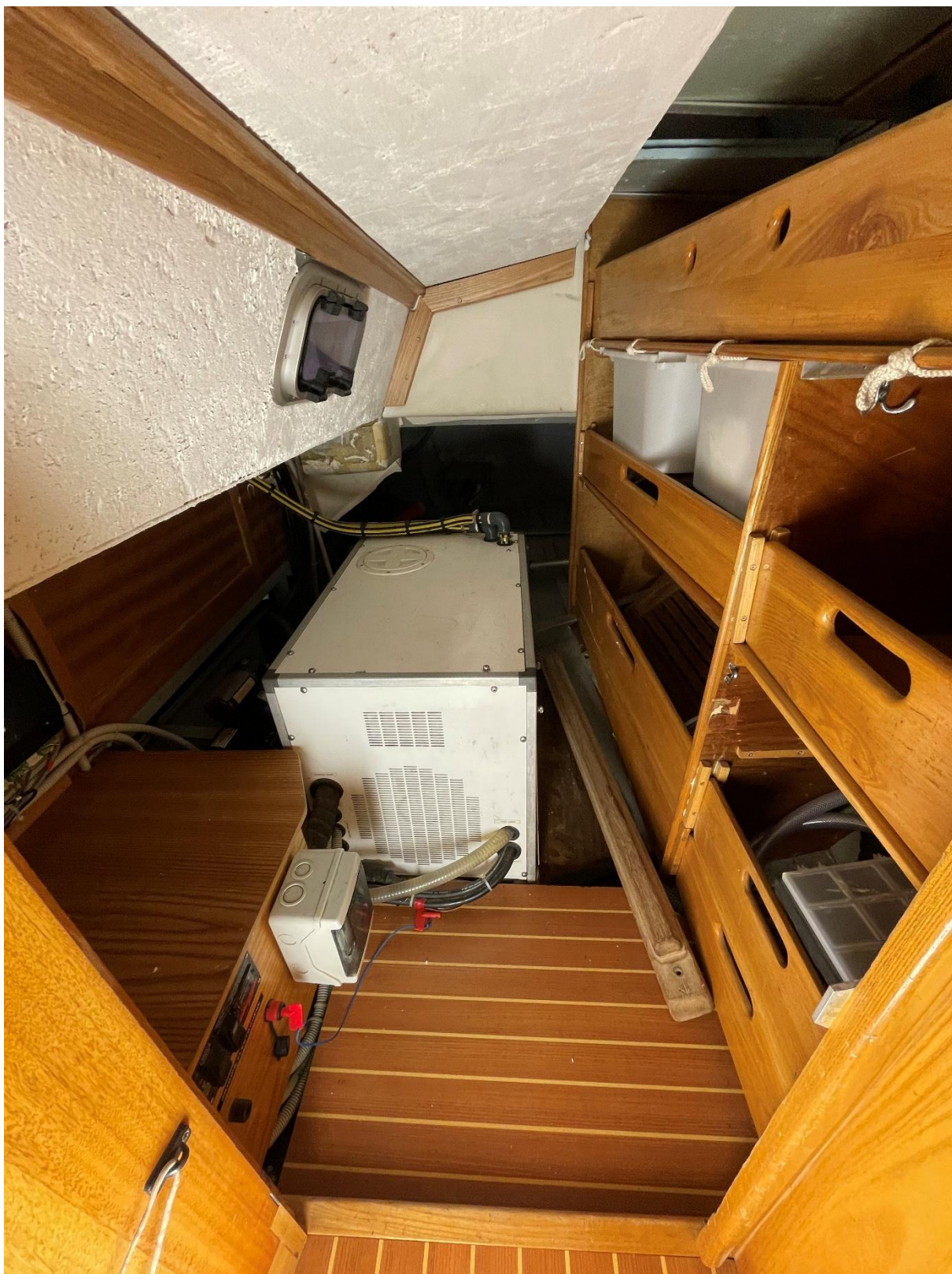
OVNI 435 – Aft portside technical room
